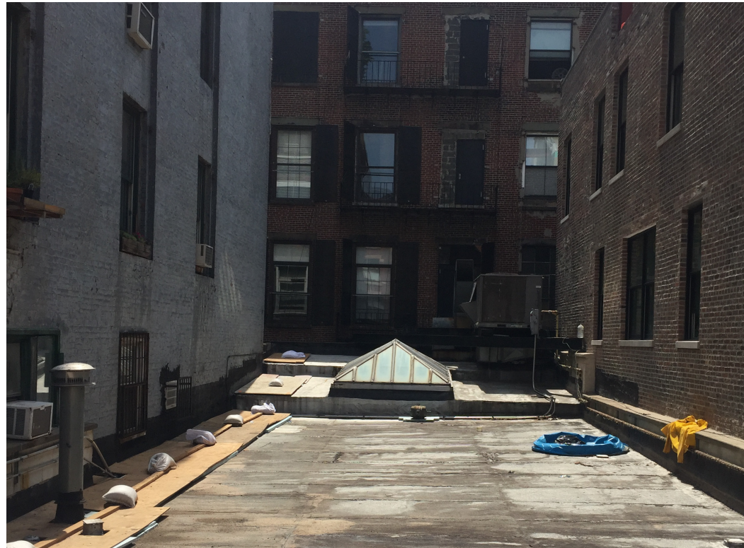
EXISTING ROOF LOOKING EAST
